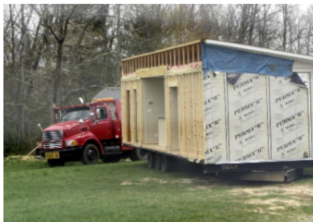
Figure 2. A mobile home being prepared for transport. Source: Andy Melton (trekkyandy), https://www.flickr.com/photos/trekkyandy/2402946311/
